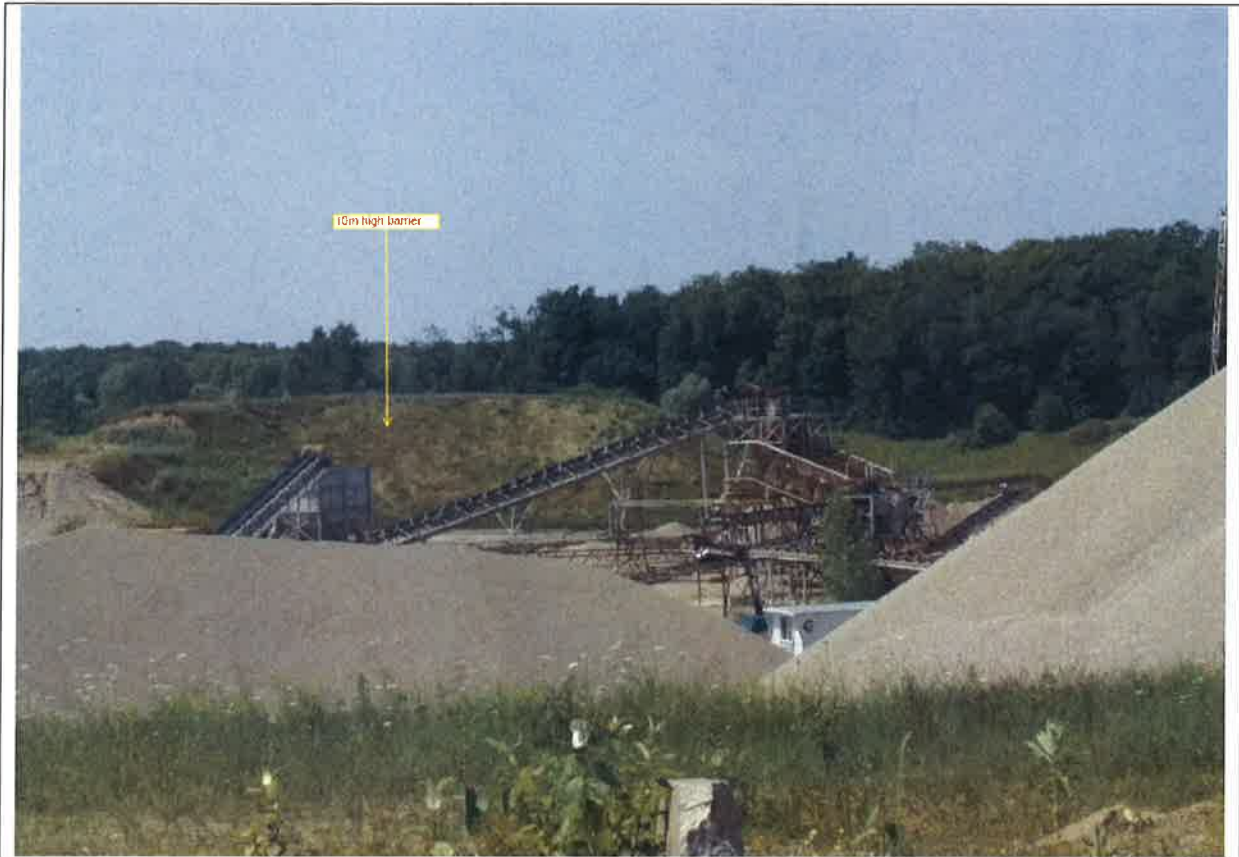
FIGURE 3: 10 METER HIGH BERM AT PROCESSING PLANT
