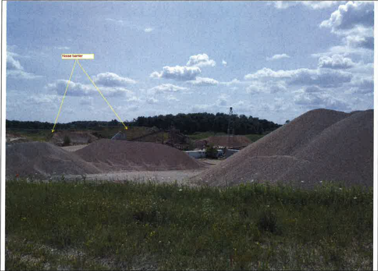
FIGURE 2: BERM AND STOCKPILES SURROUNDING PROCESSING PLANT
